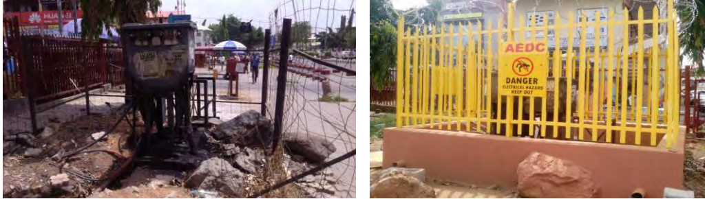
Picture 1: Before & After Picture of Banex Plaza Distribution Substation, Wuse 2 Abuja
